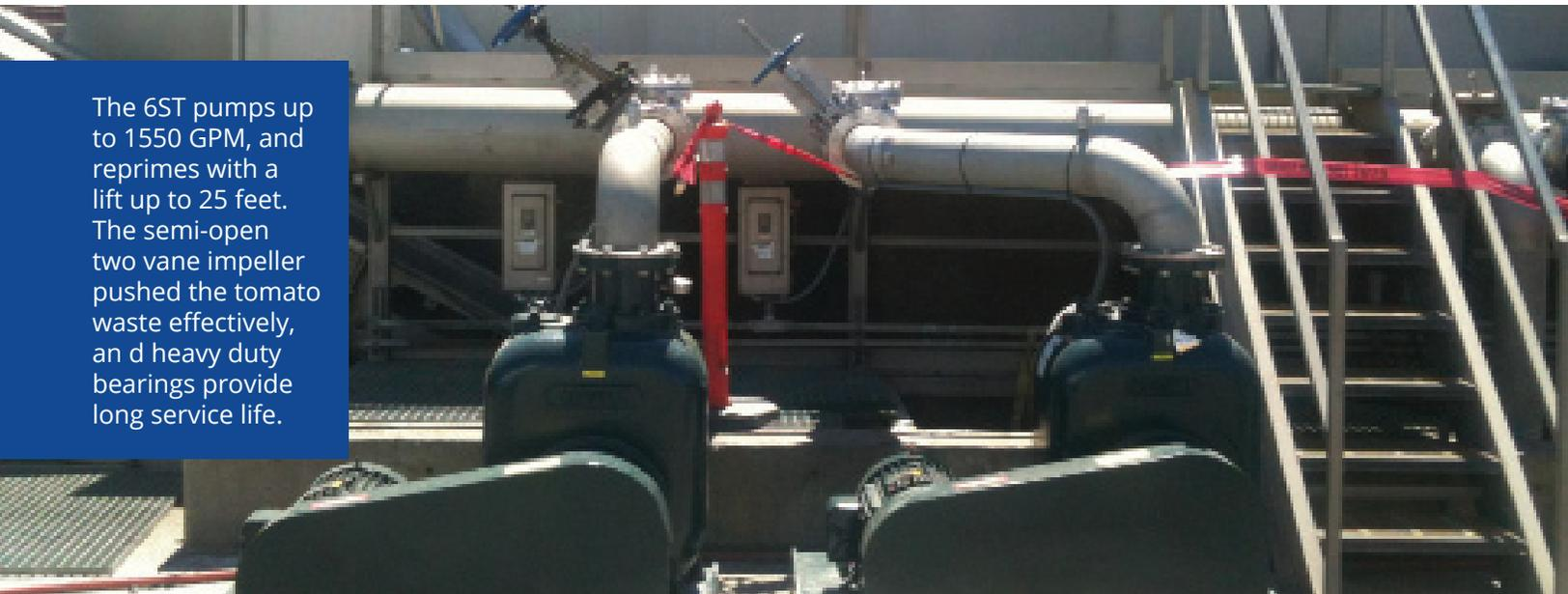
The 6ST pumps up to 1550 GPM, and reprimers with a lift up to 25 feet. The semi-open two vane impeller pushed the tomato waste effectively, and heavy duty bearings provide long service life.
