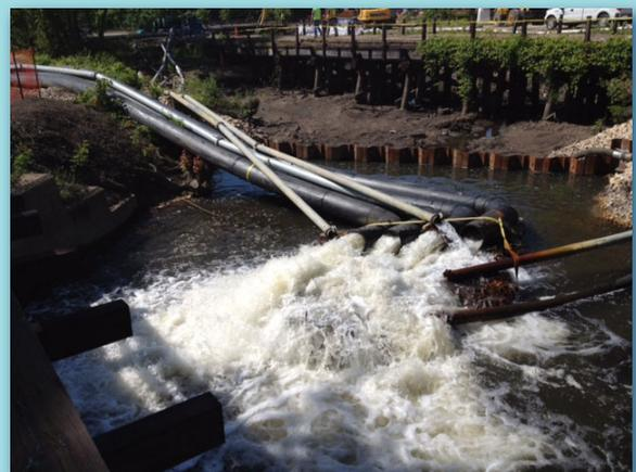
*Downstream from the contaminated soil site, the water is returned to the creek.*
