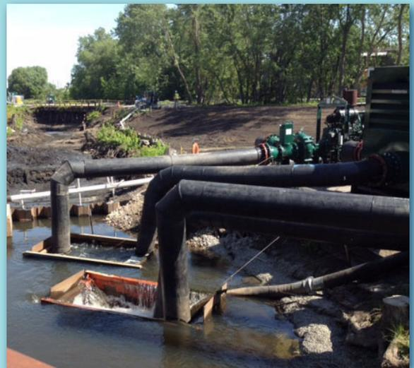
*Water is pumped from Portage Creek just upstream from the remediation area.*
