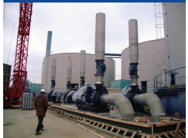
VERTICAL DISCHARGE LINES EXCITING THE PUMP STATION
