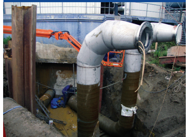
CONSTRUCTING PUMP STATION WITH SUCTION LINES LEADING FROM DECANTING TANKS
