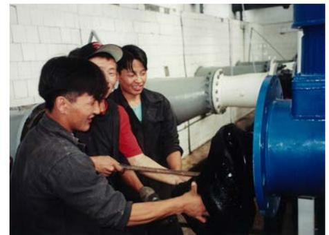
**Top:** four new Cornell Pumps in operation after installation in Mongolia. **Above:** removing a tire from the impeller when the solids screen was bypassed in the initial start up of the pumps.
